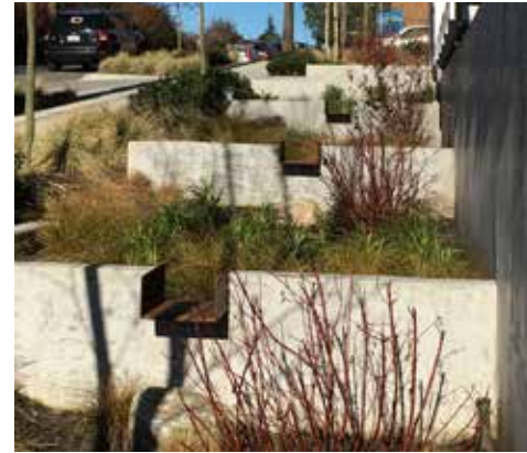
Bioretention Planter Wall
