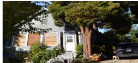
1. VIEW OF 2436 NW 56TH ST
