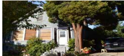
1. VIEW OF 2436 NW 56TH ST
