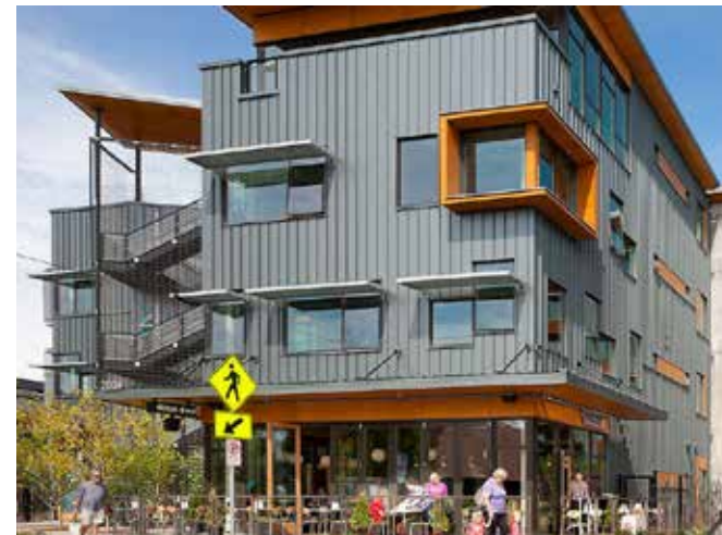
MATERIALS & ROOF EDGE.
