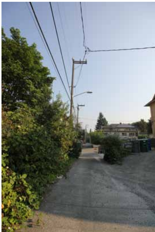
7. POWER LINES AT ALLEY
