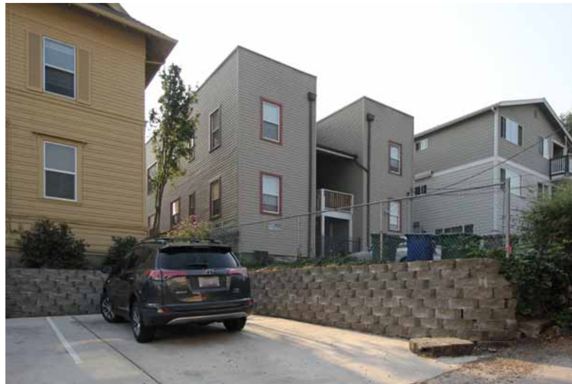
8. DROP IN GRADE NORTHWEST OF PROPERTY LINE
