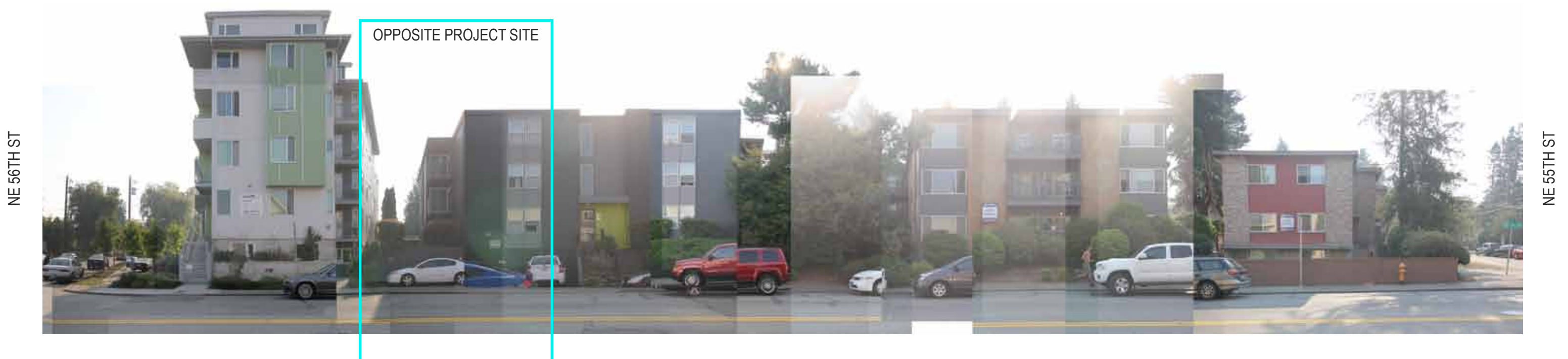
15TH AVE NE: LOOKING EAST - OPPOSITE PROJECT SITE
