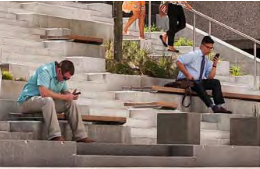
Concrete Steps with Integrated Woodtop Seating
