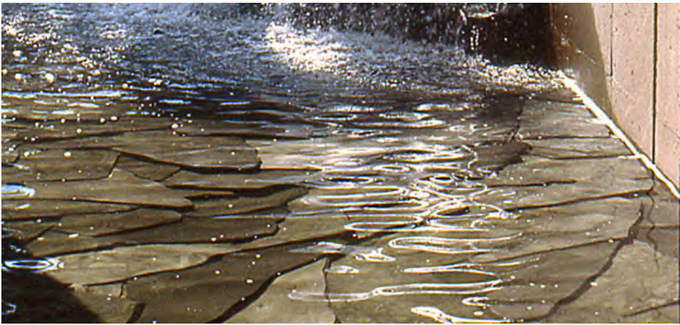
Shiplapped Slate on Water Feature Bottom for Winter Effect
