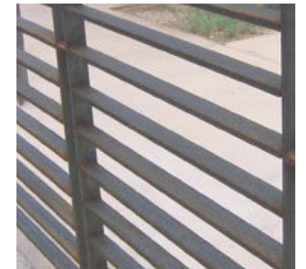
④ OPEN METAL RAILING
