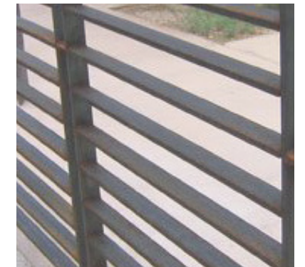
④ OPEN METAL RAILING
