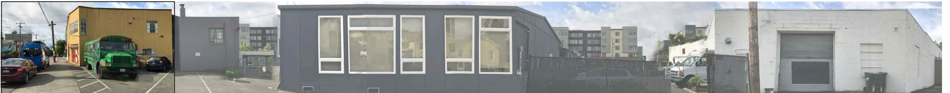
ACROSS FROM SITE
