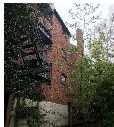
Facing northeast from north side yard. View of 1005 Apt metal fire escape, blank 1st floor walls, and top of fence.
