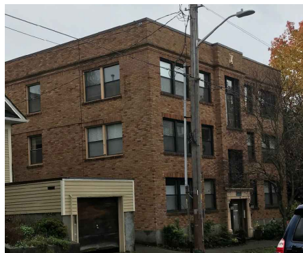
(B) Brevard Apartments - 3-story brick
