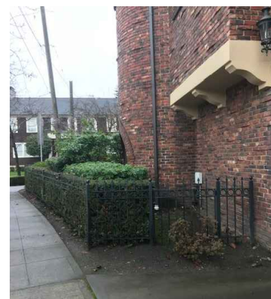
Facing north from sidewalk on 10th Ave E. Looking at courtyard on street in front of 1005 Anhalt Apartments.
