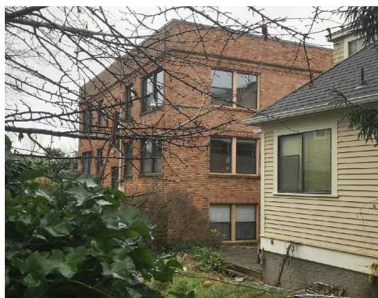
Facing southwest from back yard. Facing 620 10th Ave E and Brevard Apts.
