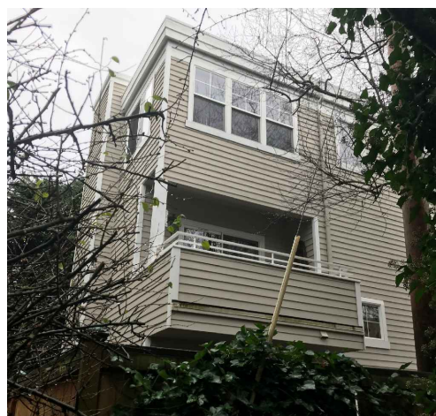
Facing southeast corner of site, looking at townhouse at 617 Federal Ave E.
