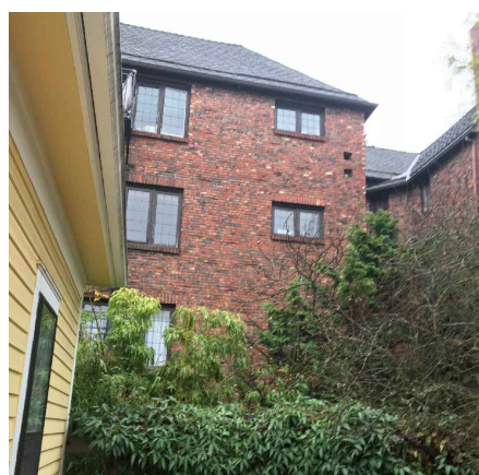
Facing north at back of house. View of 2nd to 4th floor windows on 1005 Apts.
