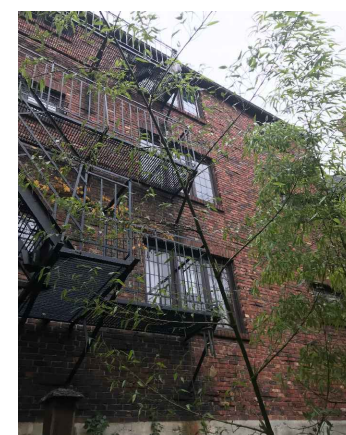
Facing north from north side setback. View of 1005 Apt metal fire escape, upper windows and bamboo.
