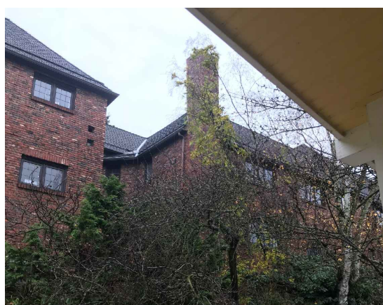
Looking at the northeast corner from back porch. Facing small courtyard and chimney of 1005 Apts.
