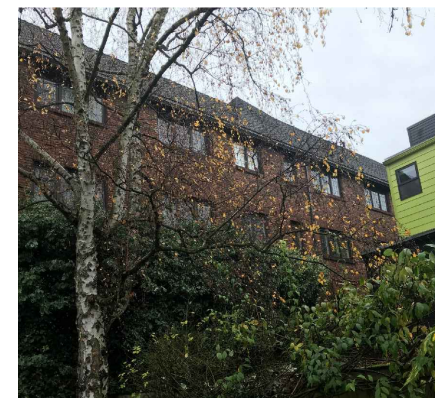
View at rear of property facing northeast. Looking at 1005 Apts & Fedroy Apts.
