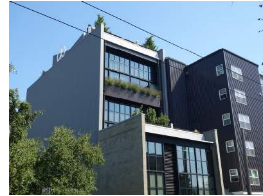
New Contemporary Construction on QA Ave
