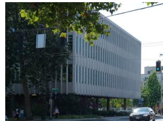
Modern office building with simple fenestration
