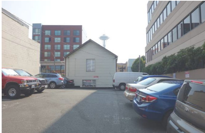
1: Rear of Site - Looking east
