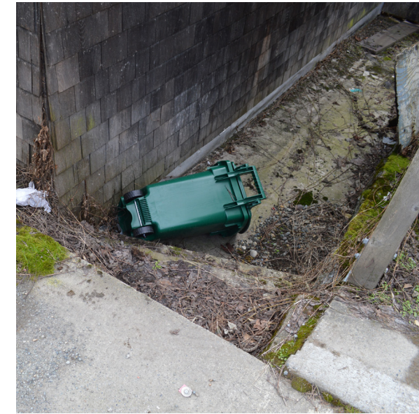
5. EXISTING PARCEL B, NORTHEAST PROPERTY CORNER
