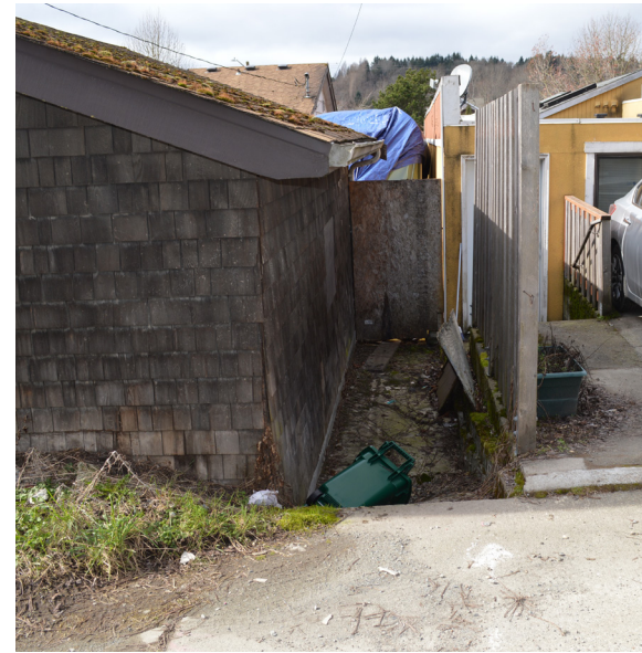
5. EXISTING STRUCTURE AND PARCEL B, NORTHEAST PROPERTY CORNER
