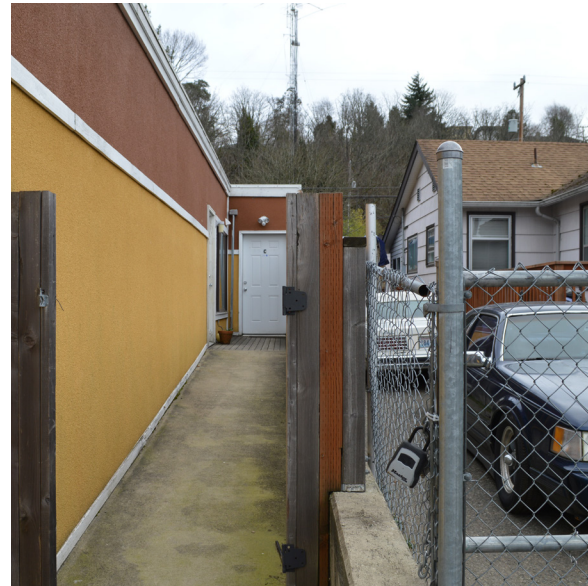
1. PARCEL A, NORTHWEST PROPERTY CORNER
