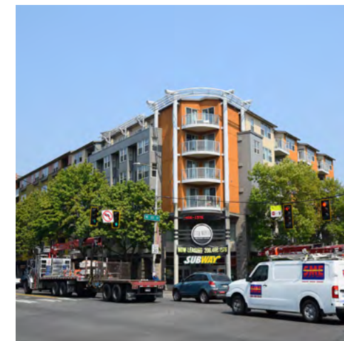
14. City North Seattle Apartments
