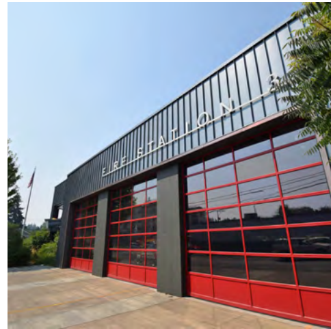
1. Seattle Fire Station 39
