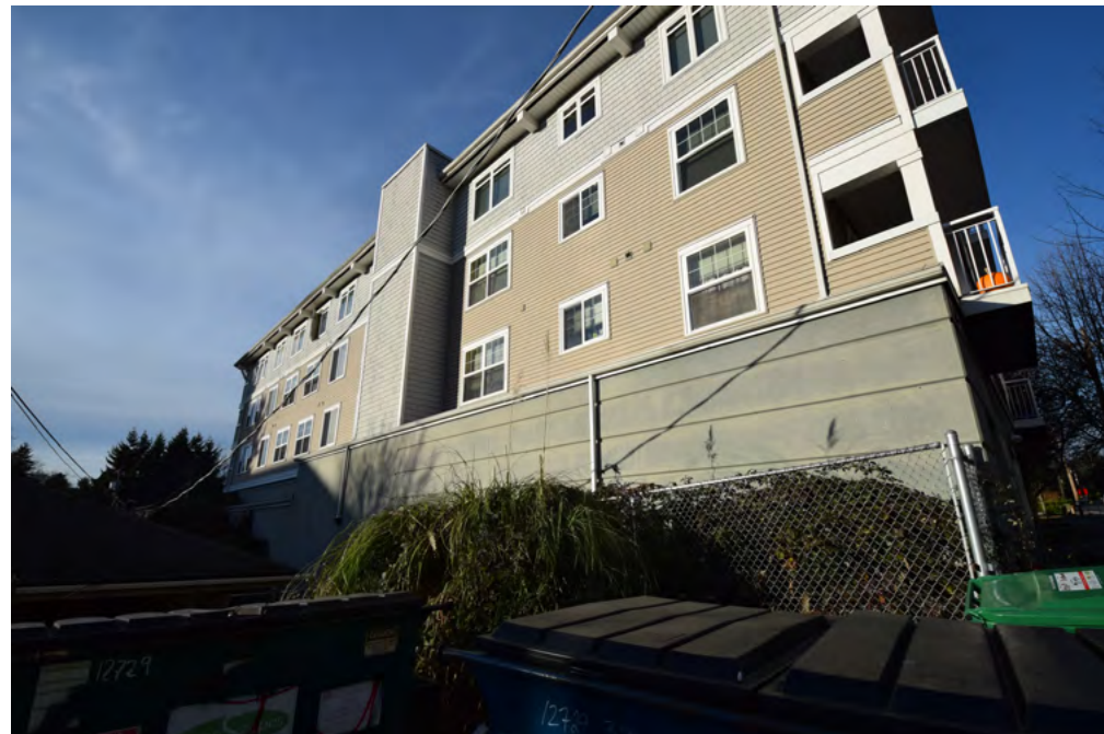
4. View from northeast corner of lot, looking towards northern neighboring building. Apartments can be seen set back approximately 5' from lower level.
