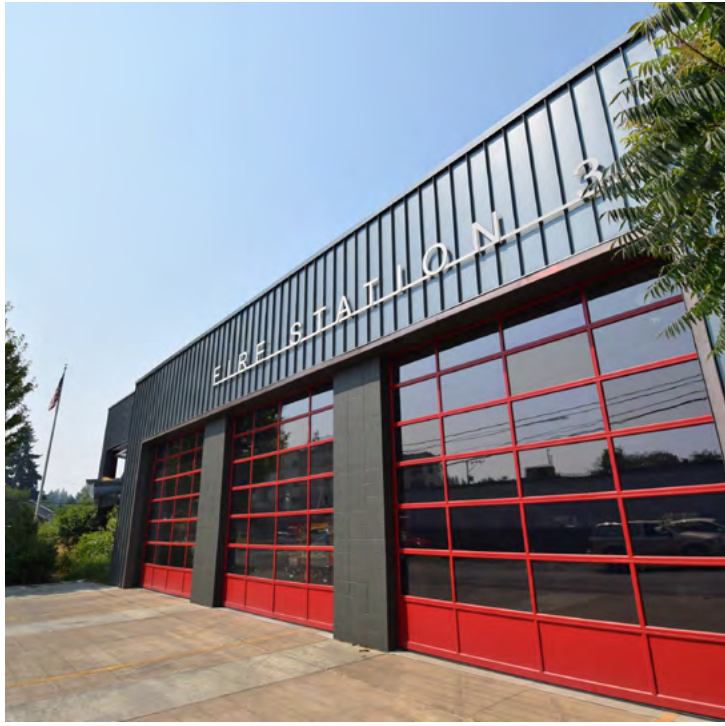
1. Seattle Fire Station 39
