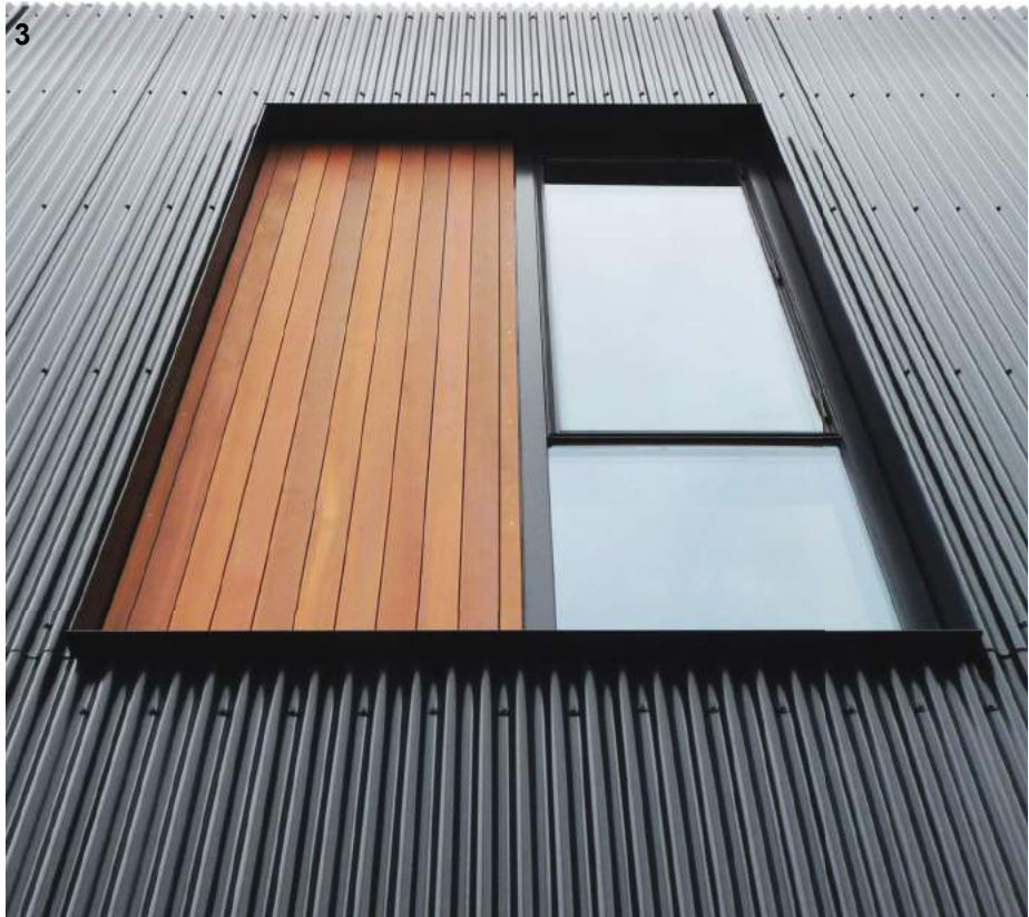
MATERIAL PRECEDENT - WINDOW GROUPING TRIMMED WITH LOW-PROFILE FLASHING
