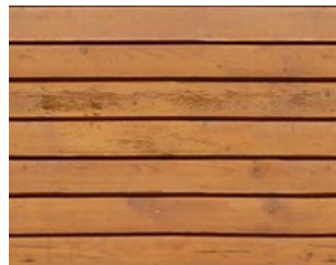
CEDAR SIDING AT EAVES AND FINS
