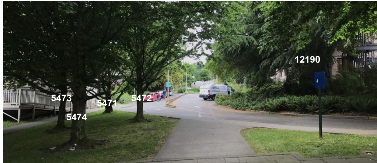
Existing trees to be removed as part of building construction, C8 parking lot demolition, pedestrian and accessibility improvements.
