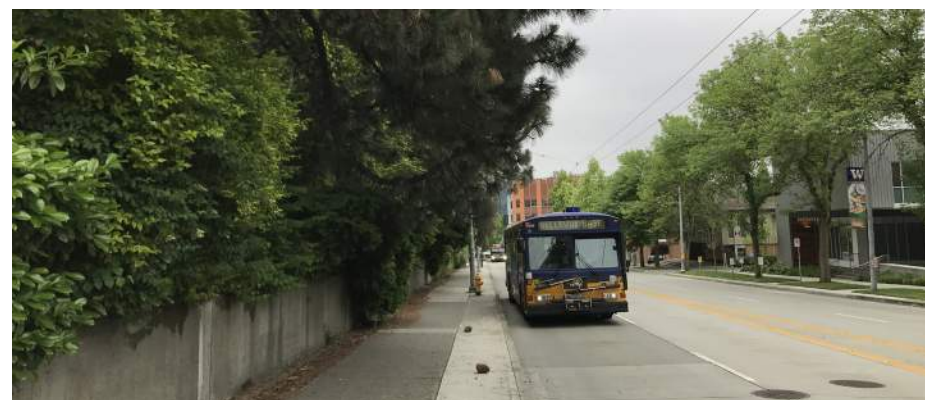
15th Ave Existing Photos
