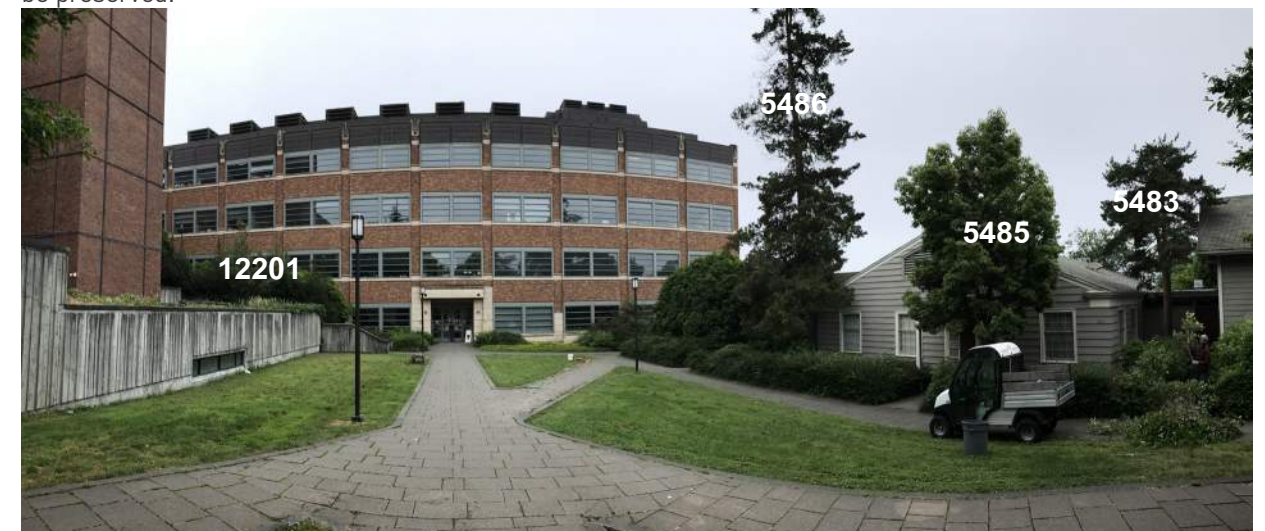
Guthrie Annex 01 on the right hand side to be demolished.
