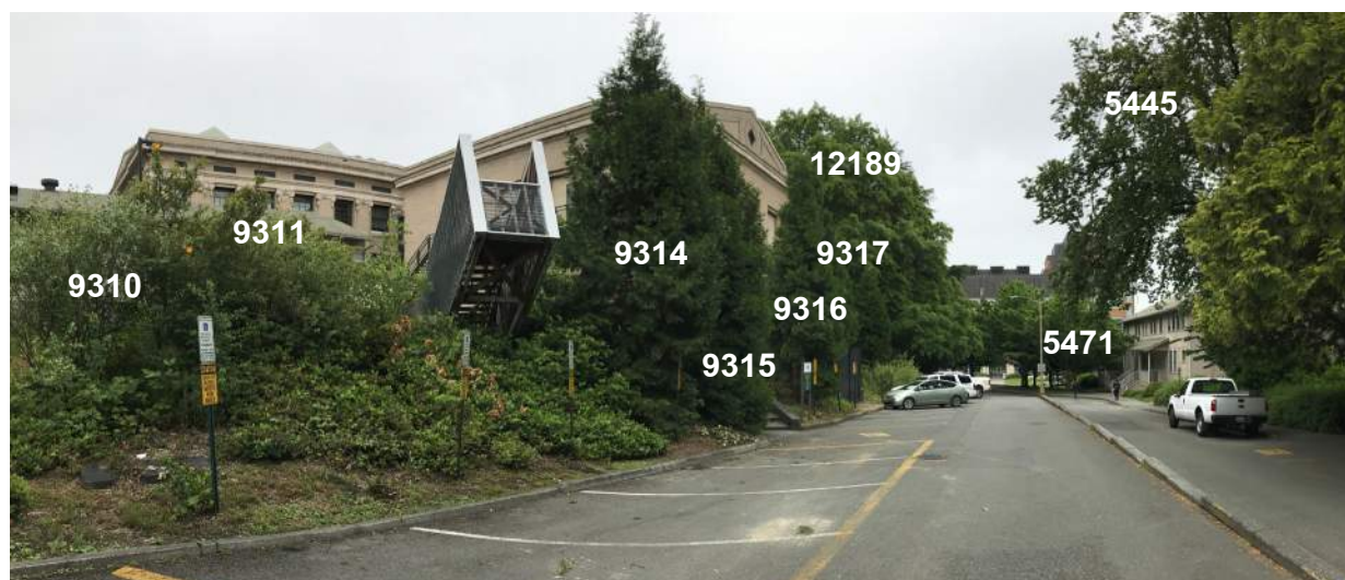
Existing C8 parking lot to be demolished for building construction and to create a pedestrian oriented, ADA accessible route. Existing tree #12189, an exceptional Water Oak to be preserved, is visible in the background.
