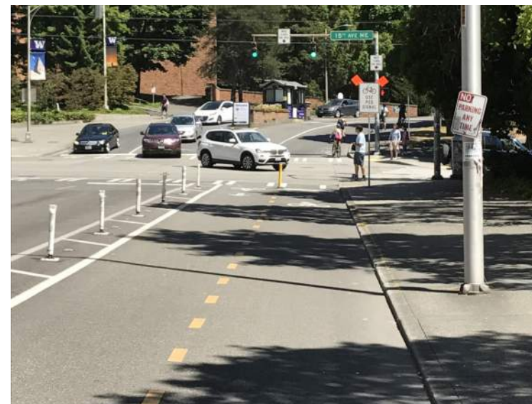
(3) Existing two-way protected bicycle lanes on NE 40th St.
