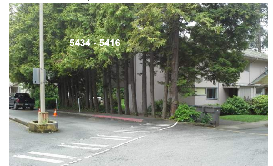
C8 parking lot, existing trees and Guthrie Annex 03 to be demolished for building construction.
