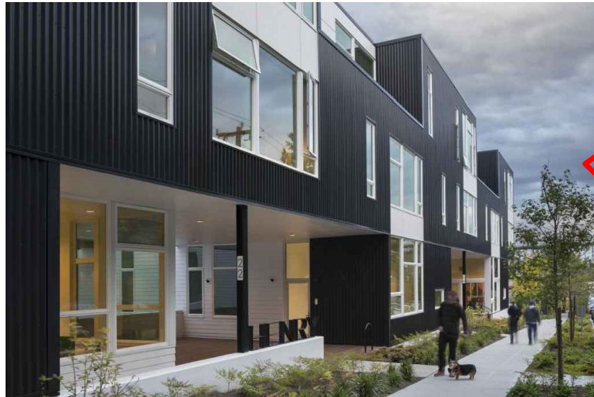
CORRUGATED BLACK METAL SIDING ON WHITE WINDOWS (NARROW CORRUGATION)+ HARDIE PANEL INSERTS
