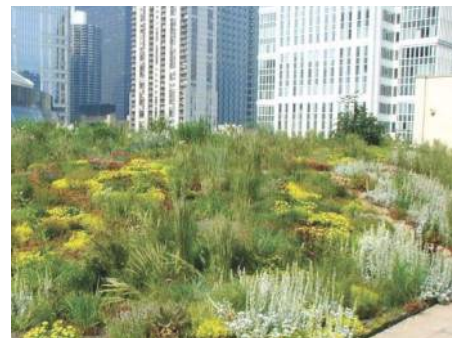
Green Roof planting manages stormwater
