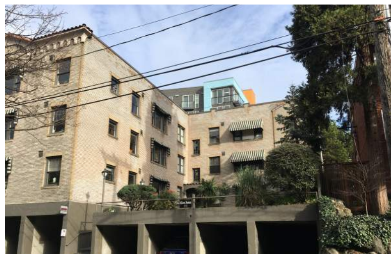
8. 512 BOYLSTON AVE | STREET COURTYARD
