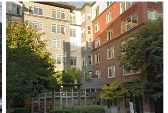
7. 1610 BELMONT AVE | STREET COURTYARD
