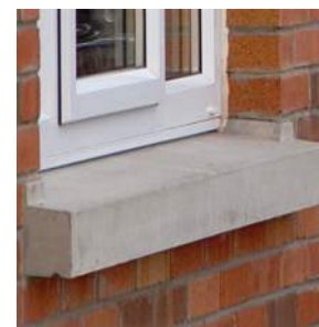
3. PRECAST CONCRETE SILL COLOR TO MATCH CASTLE GRAY BRICK.
