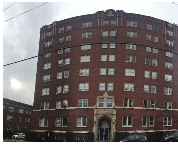
2 BELMONT AVE LOOKING WEST
