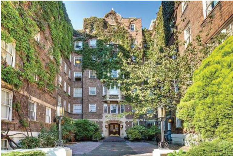
5. BILTMORE APTS. | STREET COURTYARD
