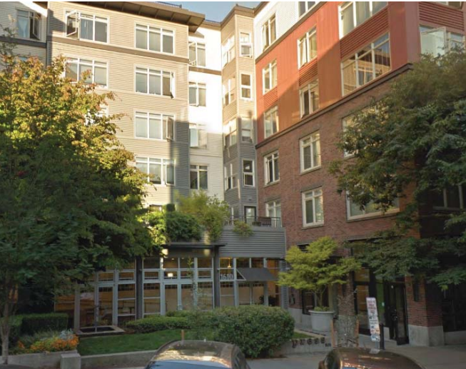
7. 1610 BELMONT AVE | STREET COURTYARD
