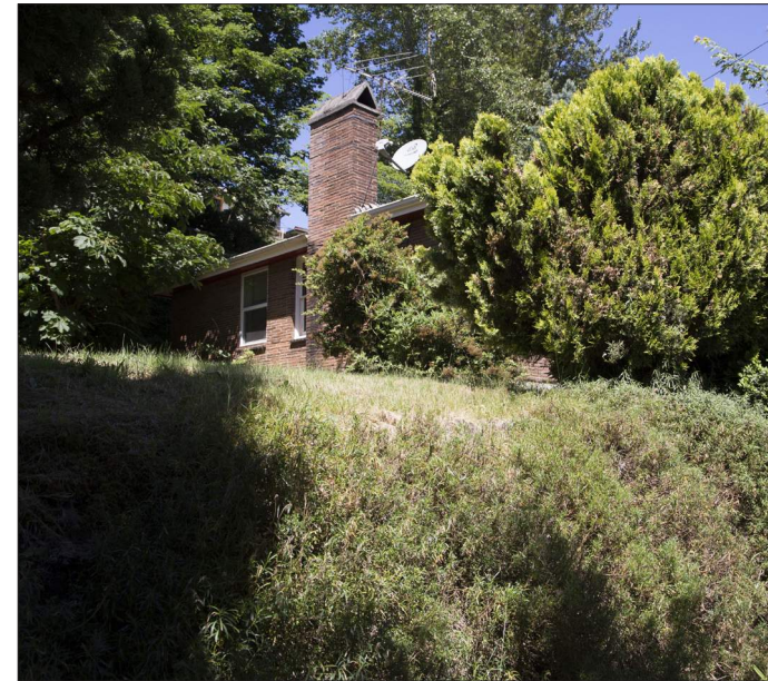
2 SOUTH VIEW OF SITE
