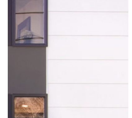
④ HARDIE PANEL (BETWEEN WINDOWS)
