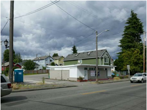
VIEW FROM SW
