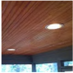
① RECESSED CAN LIGHTS (SOFFIT)
