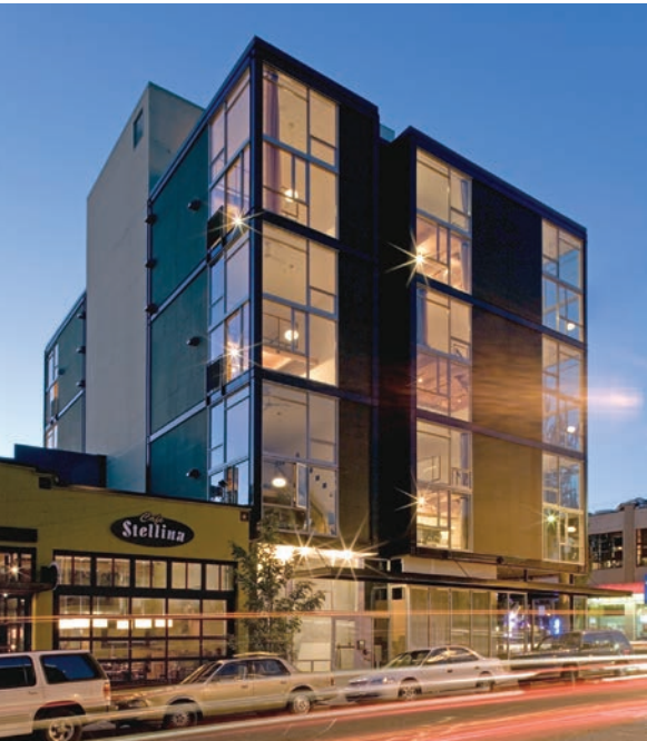
4 Variation to the window patterning creates visual interest within a simple material palette
