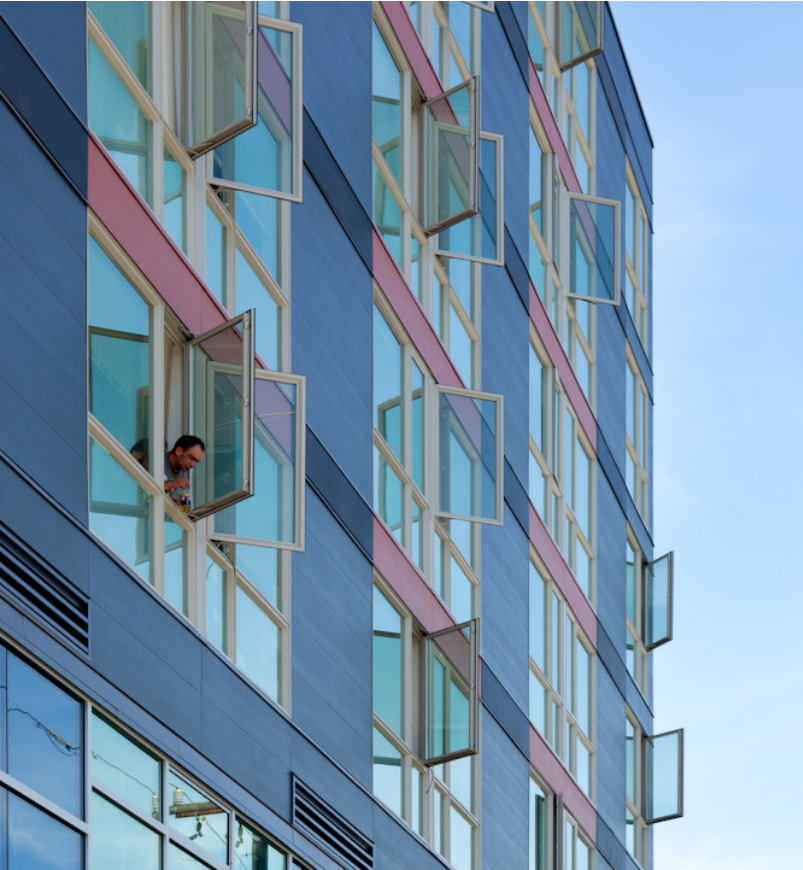
2 Facade patterning considers and integrates the unit venting strategy to minimize the visual impact
