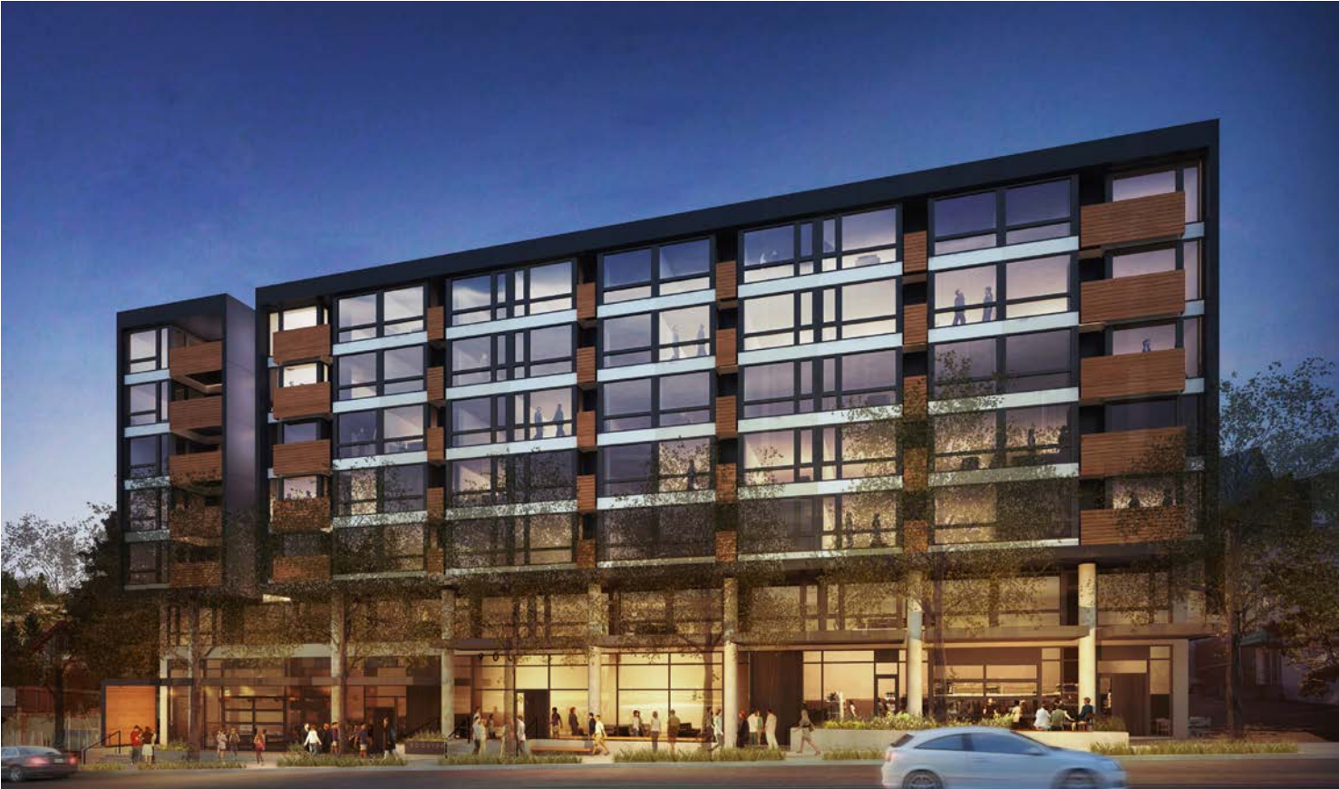
1 Window heads meeting the ceiling maximize natural light in the units and lighten the massing of larger buildings.
