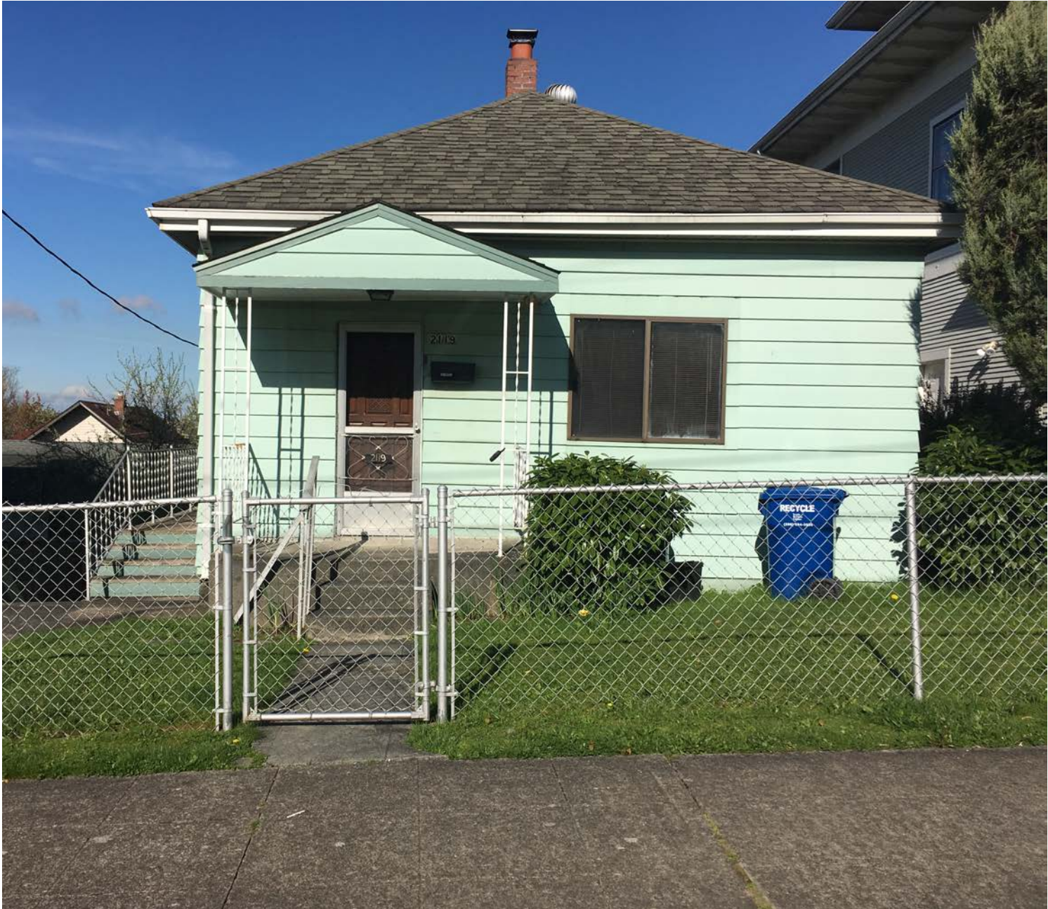
5. front / east facade of existing residence
