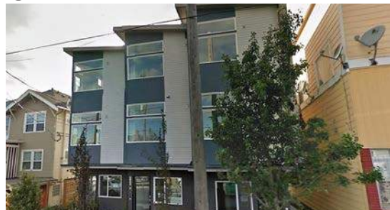
15 Townhouses one block east, off 14th Ave S
