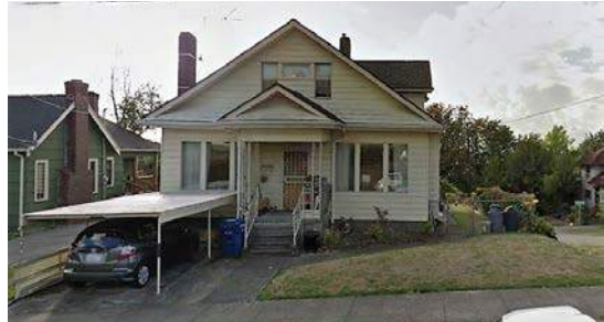
1 Single family home off 13th Ave S and S. Walker St.
