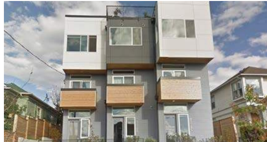
7 Townhouses on 13th Ave S across from site
