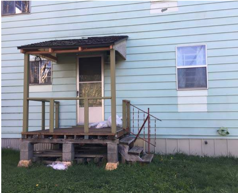
4. rear (west) facade and deck / existing structures
