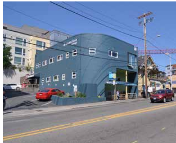
④ Recessed entry along NE 65th Street Commercial Use along NE 65th Street 916 NE 65th St Built: 1990
