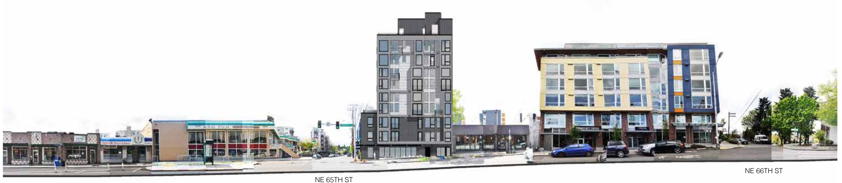
VIEW OF EAST ELEVATION ON ROOSEVELT WAY NE
