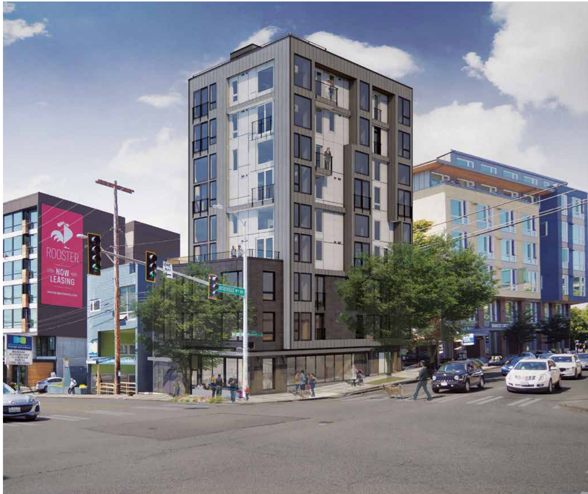
1 View looking Northwest at Corner Facades
