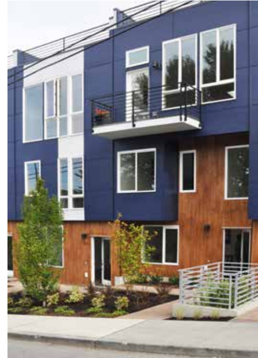
Rowhouses at 90 E Newton Street
