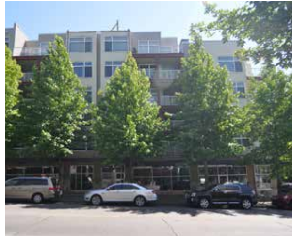
② Decks along NE 65th Street. Mixed use Apartments 6410 9th Ave NE Built: 1999, 47 units, 6 stories
