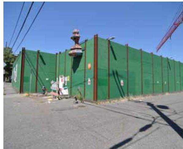
⑥ On going construction near project site Future Roosevelt Light Rail Station 6612 Roosevelt Way NE Built: Under Construction
