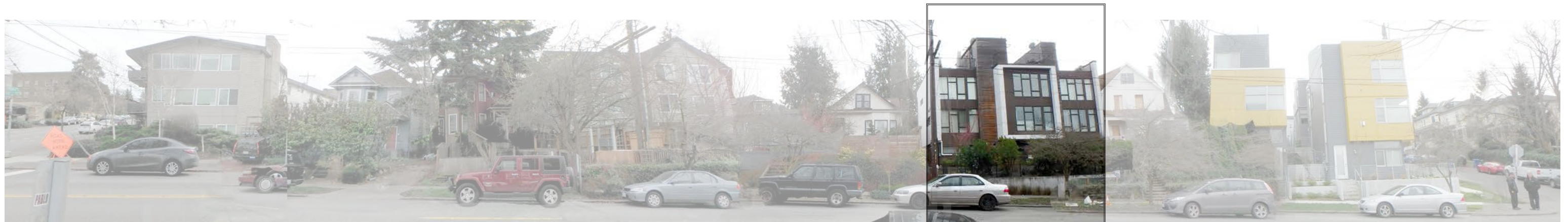
14TH AVE LOOKING EAST (B)
