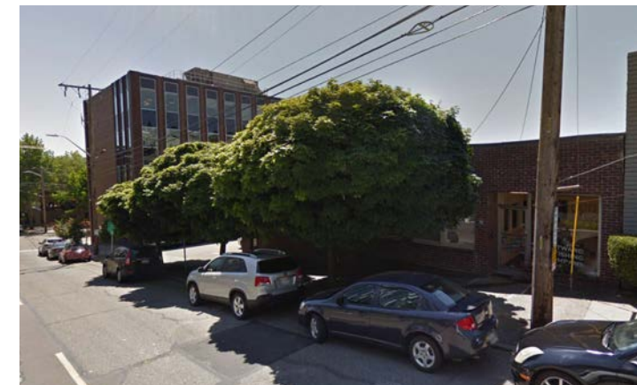
Existing Street View
