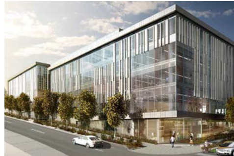
3. 450 3rd Ave W 5 Stories, Office Building
