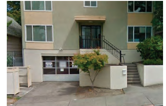
1 | Stepped, street-facing entries
