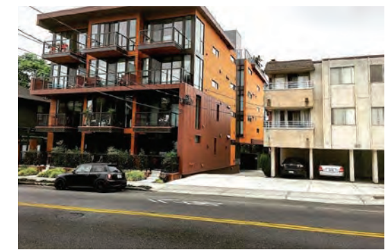
5 | Terraced outdoor decks; neighboring building
