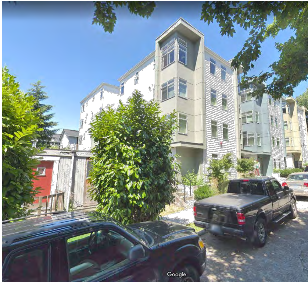
Northern neighbor; street view
