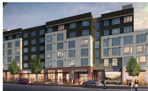
6. 419 NE 71st St 6 Stories, 130 Residential units 14,609 Sq. Ft Commercial Space 106 Parking Stalls (below grade) Construction Permit issued
