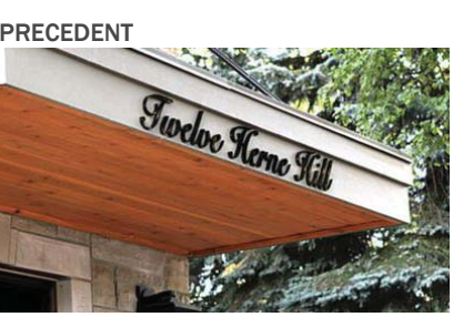
D AWNING-MOUNTED LOBBY ENTRY - STREET FACING
