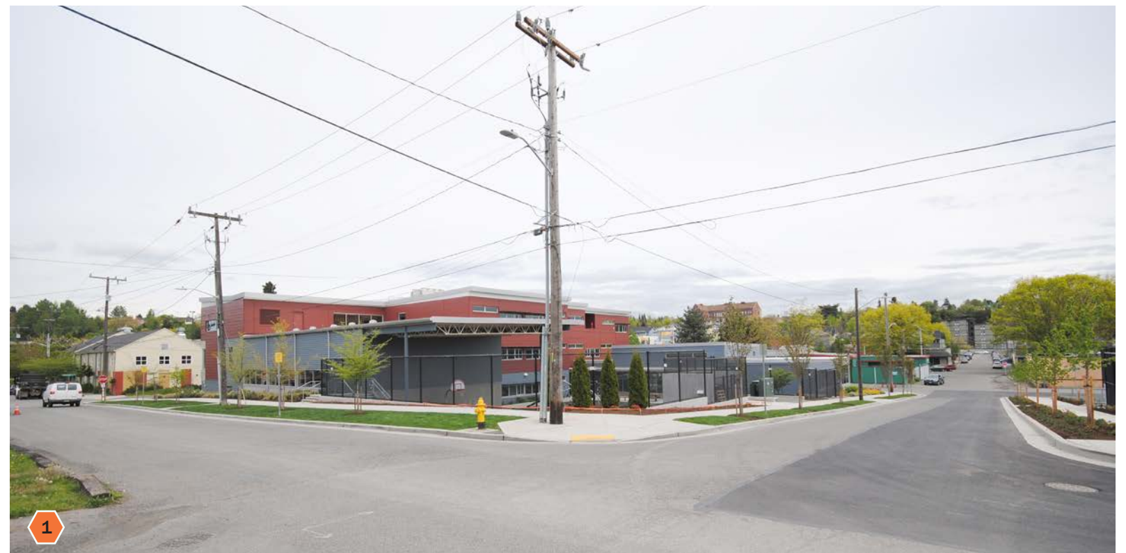
• Corner of South State Street & Valentine Place South, looking North-East.
