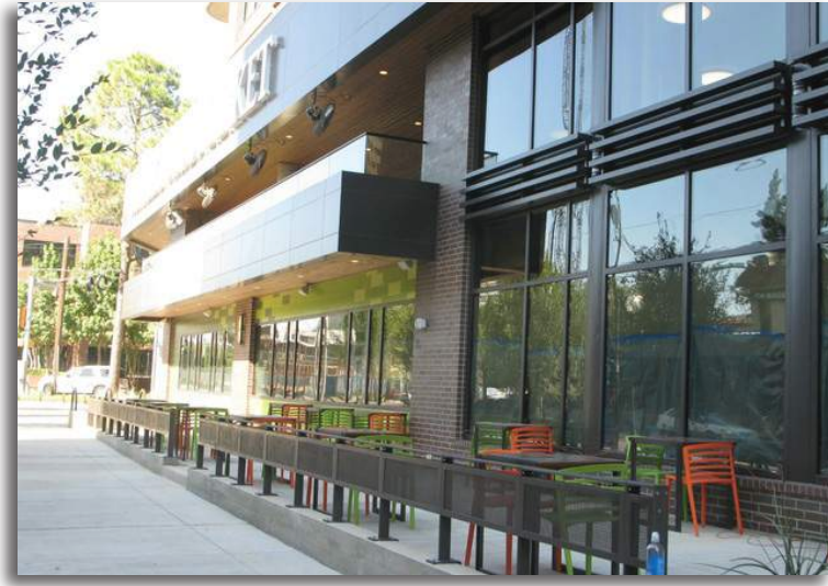
OVERHEAD PROTECTION OVER SEATING
