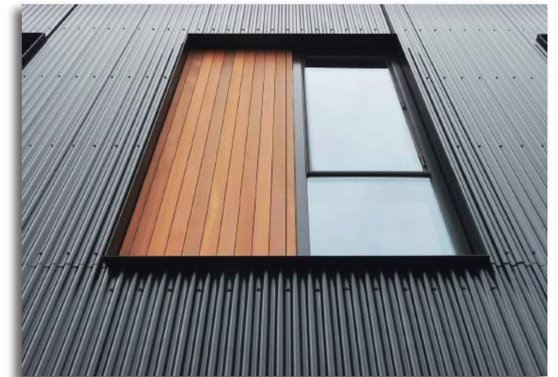
EXAMPLE OF TRIMMED WINDOW/INFILL PANEL GROUPINGS SET IN DARK METAL CLADDING
