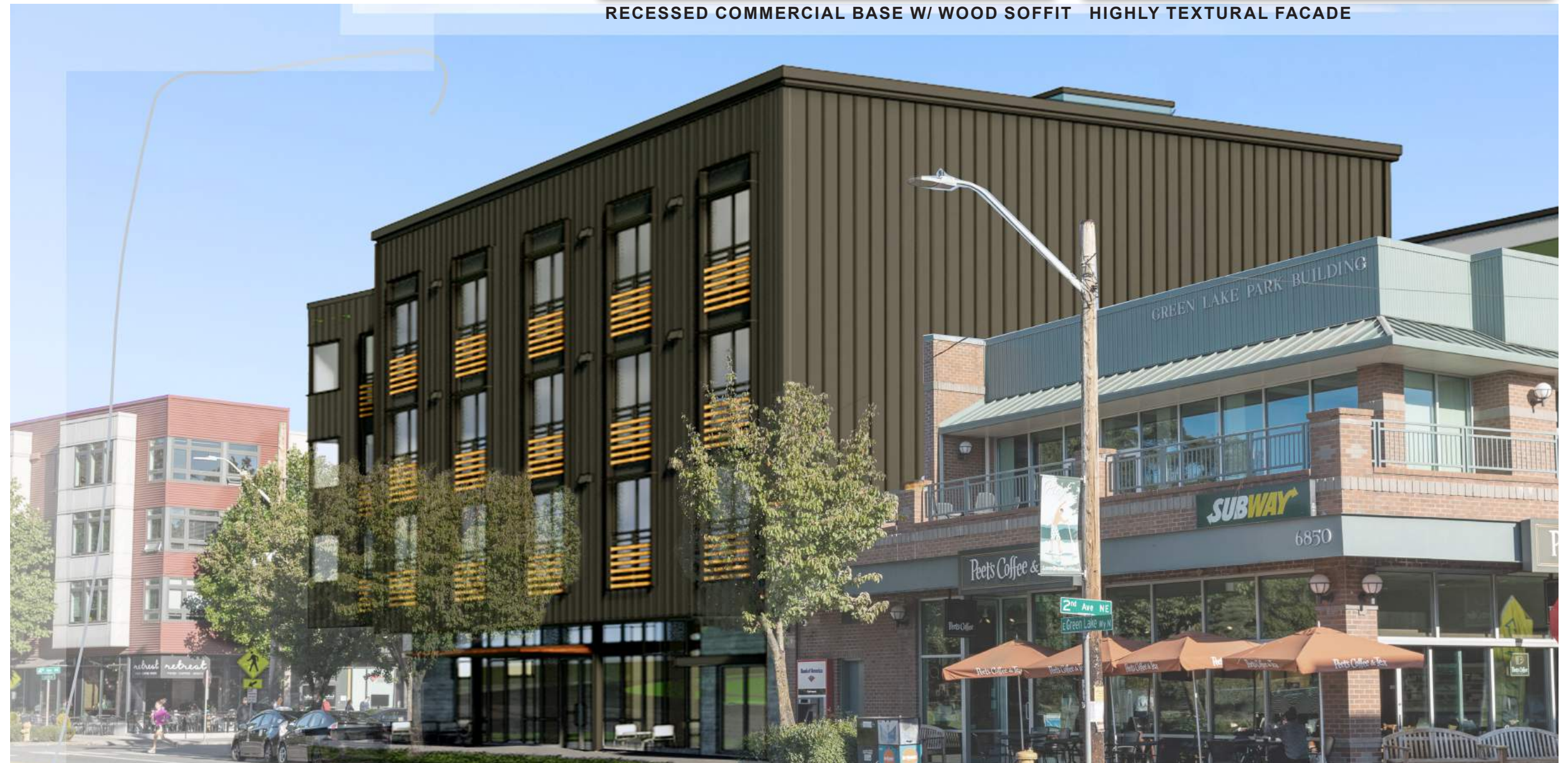
NORTHWEST CORNER VIEWED FROM EAST GREEN LAKE WAY
