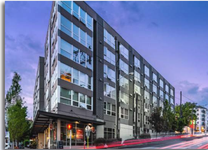
GEOMETRIC CORNER WITH WRAPPED GLAZING
