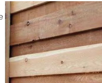
Overlapping cedar siding stained to match the wood veneer panel
