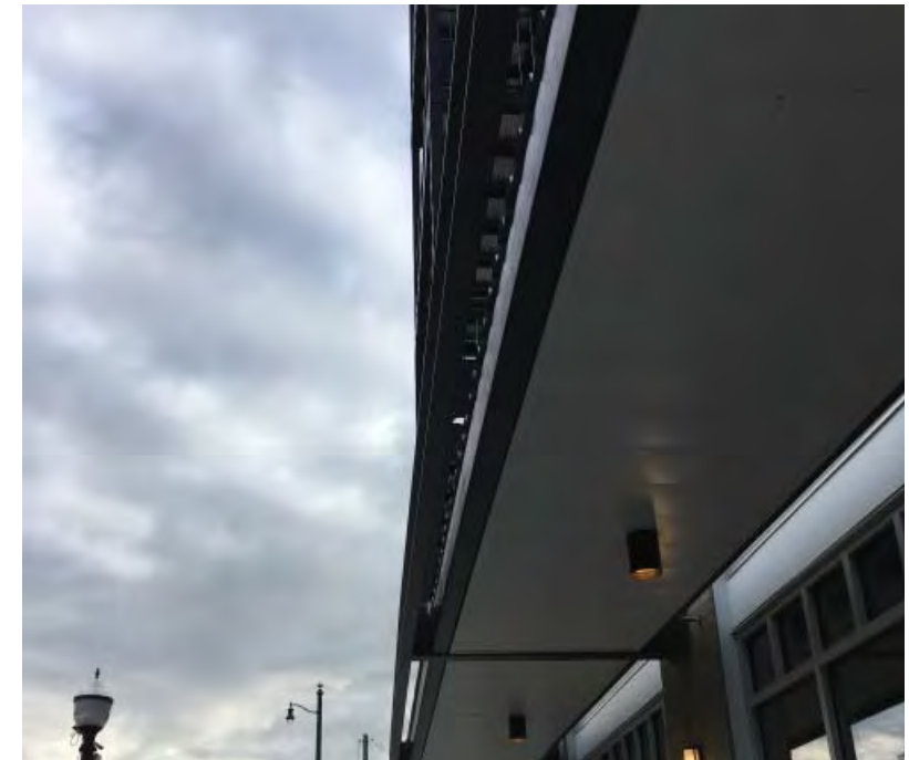
METAL CANOPY W/ SOFFIT AND DOWNLIGHTS AT MLK JR. WAY S. ENTRIES (SOFFIT TO BE BLACK)
