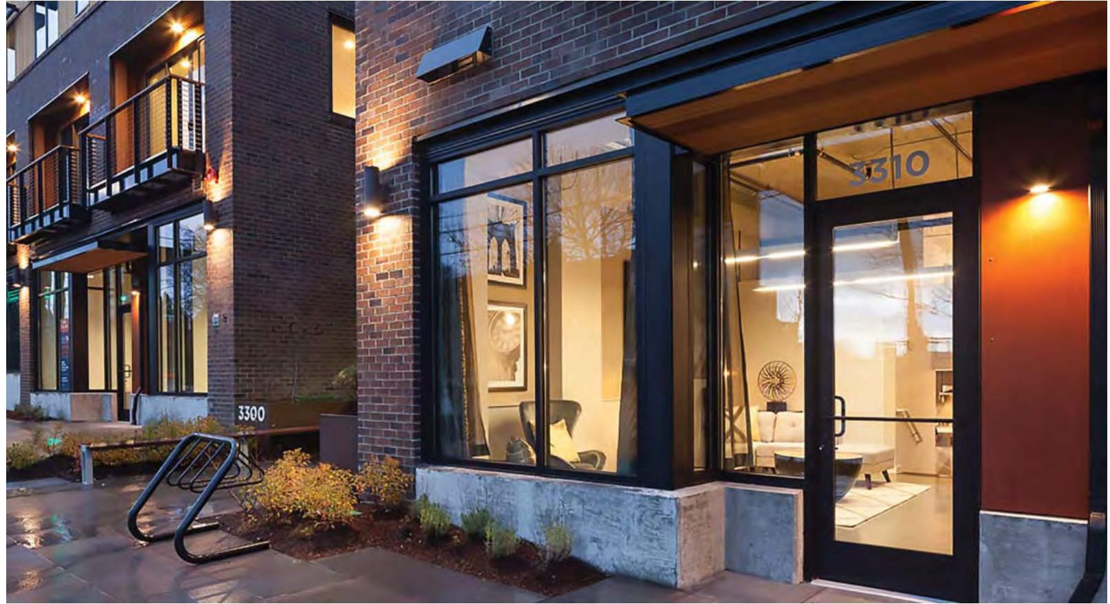
BRICK, BLACK STOREFRONT FRAMES AND CONCRETE BASE AT THE LIVE-WORK UNITS
