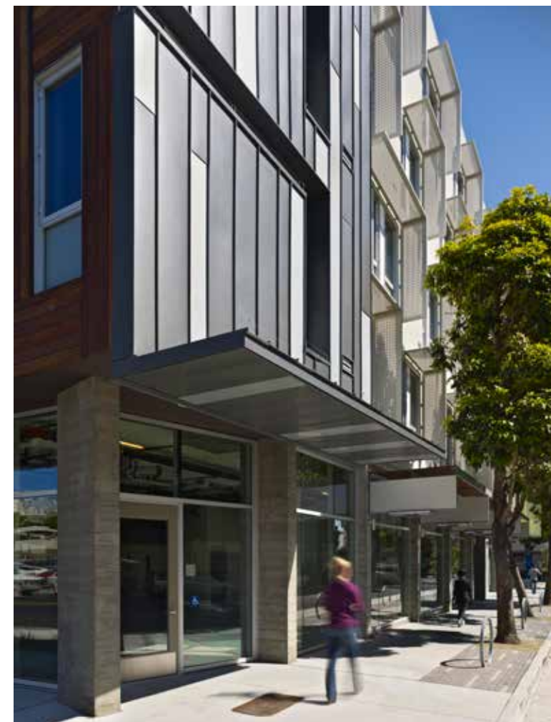
Highly transparent base helps define programmatic difference from the opaque massing above.
