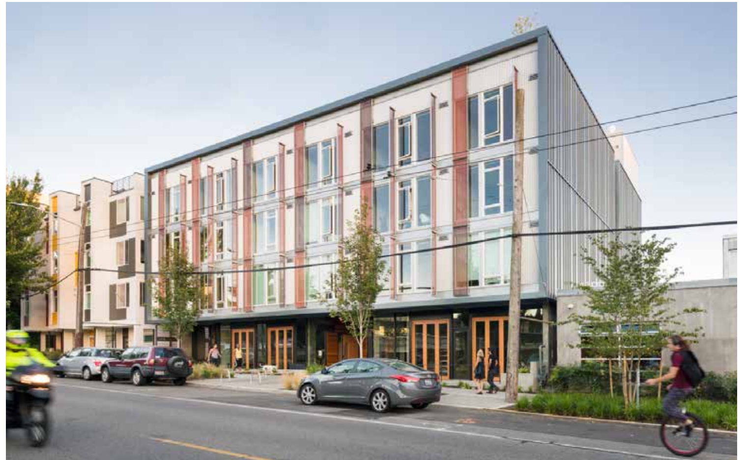
CRAFT | Mixed-Use 32-Units/, 3,500sf Retail | First Hill, Seattle | 2016 | LEED GOLD Certified
