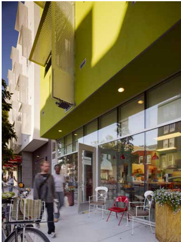
Building setback provides distinct retail expression, while serving as weather protection.
