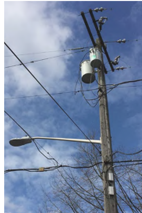
VIEW OF HVL LINE (2)
