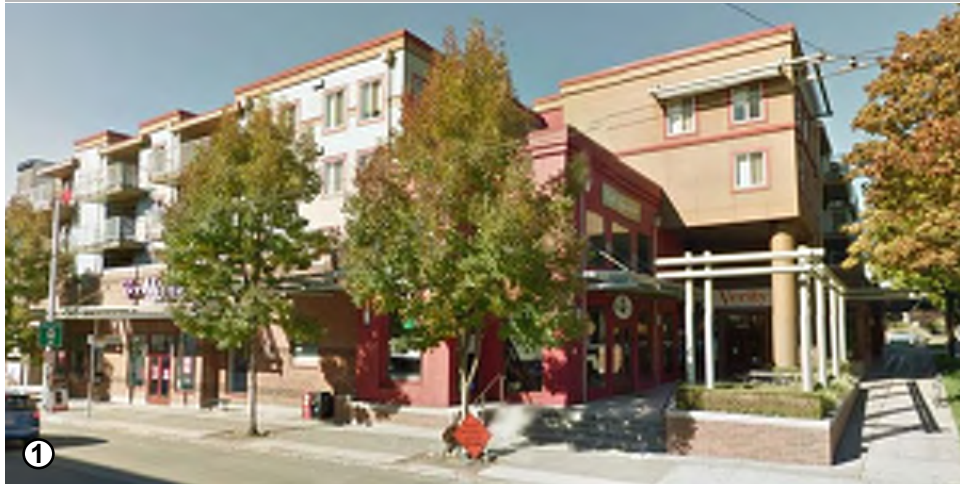
1216 N 45TH STREET Open corner to appeal to pedestrians; raised patio surrounded by landscaping creates an inviting seated space to supplement the commercial program.
