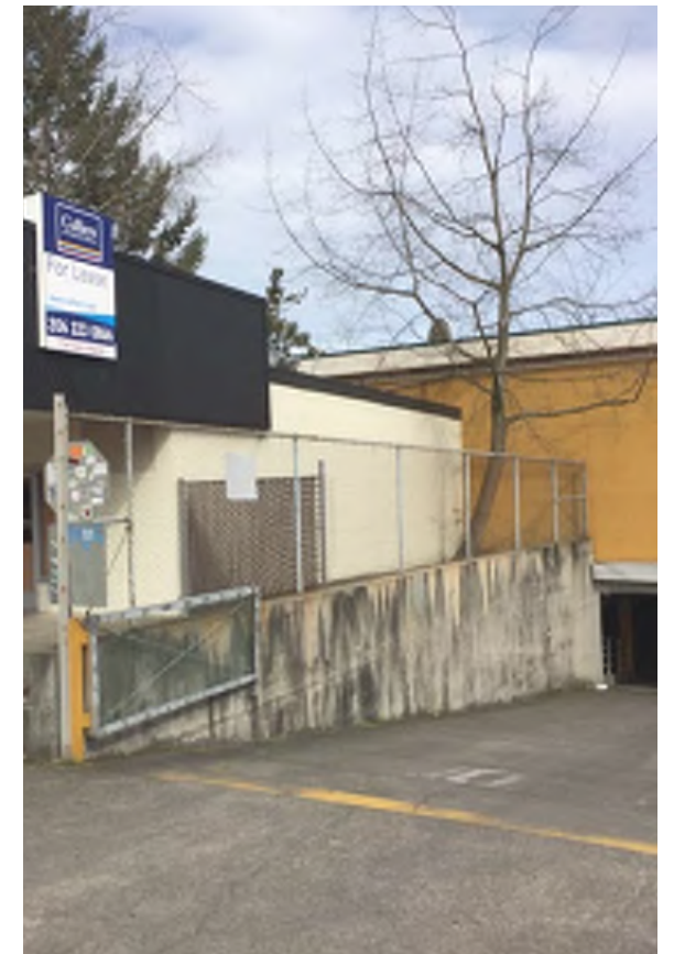
VIEW OF SOUTHERN RETAINING WALL (5)
