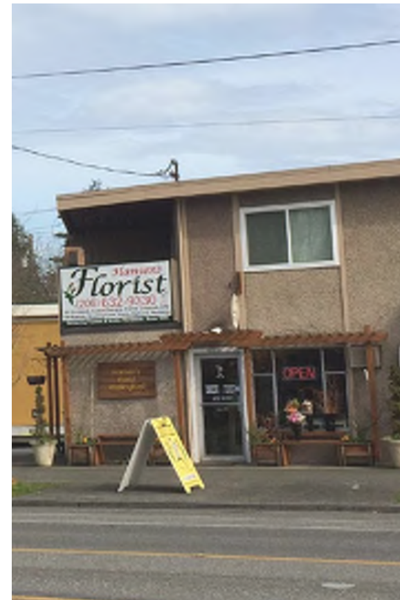
VIEW OF SOUTHERNMOST NEIGHBOR (4)
