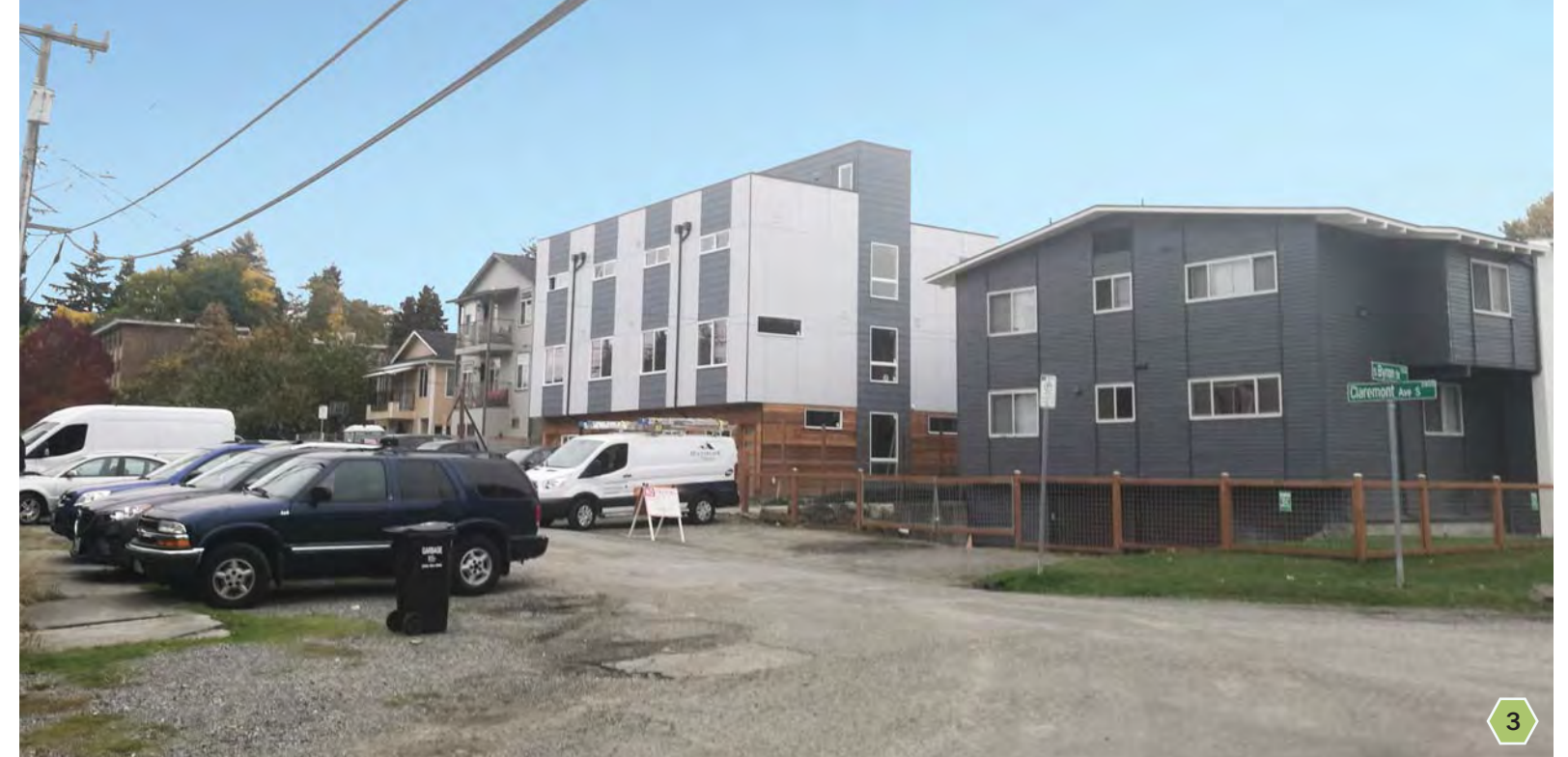
• CLAREMONT AVENUE SOUTH, LOOKING SOUTH
