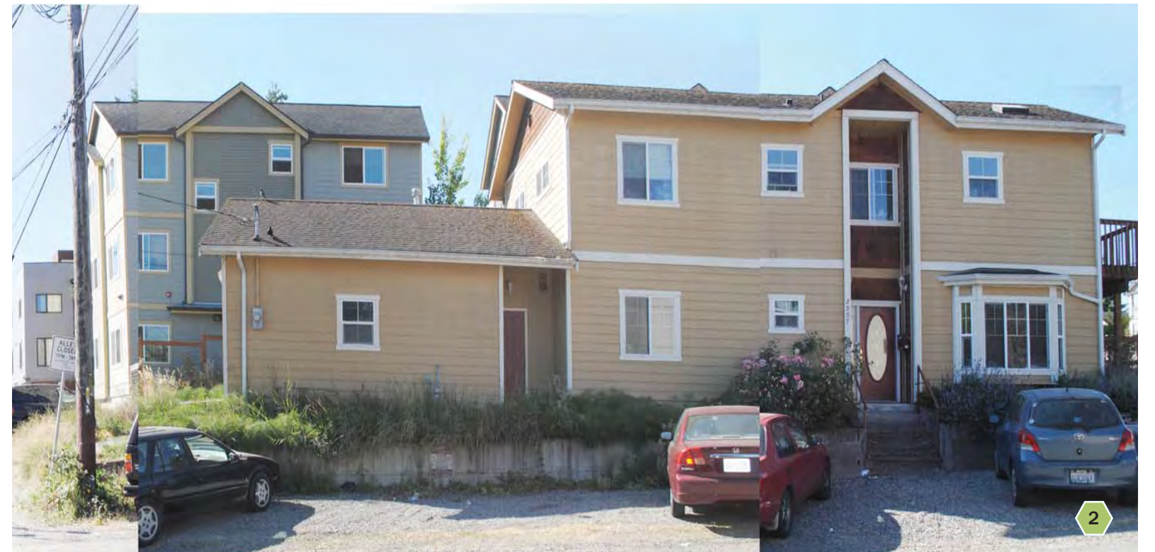
• SOUTH BYRON STREET, LOOKING SOUTH-WEST
