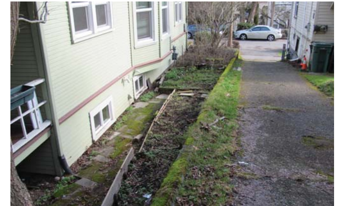
7 SOUTH PROPERTY LINE
