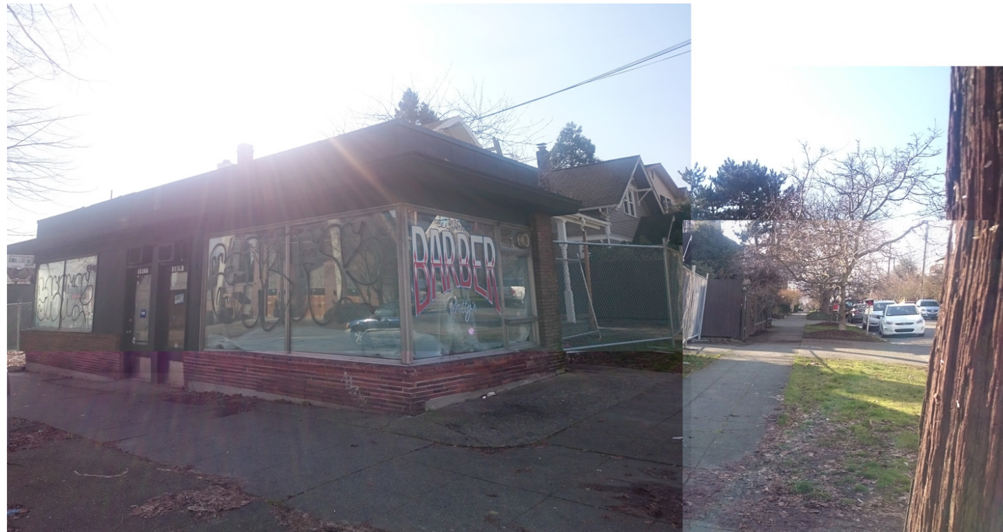
C - NORTHEAST CORNER
