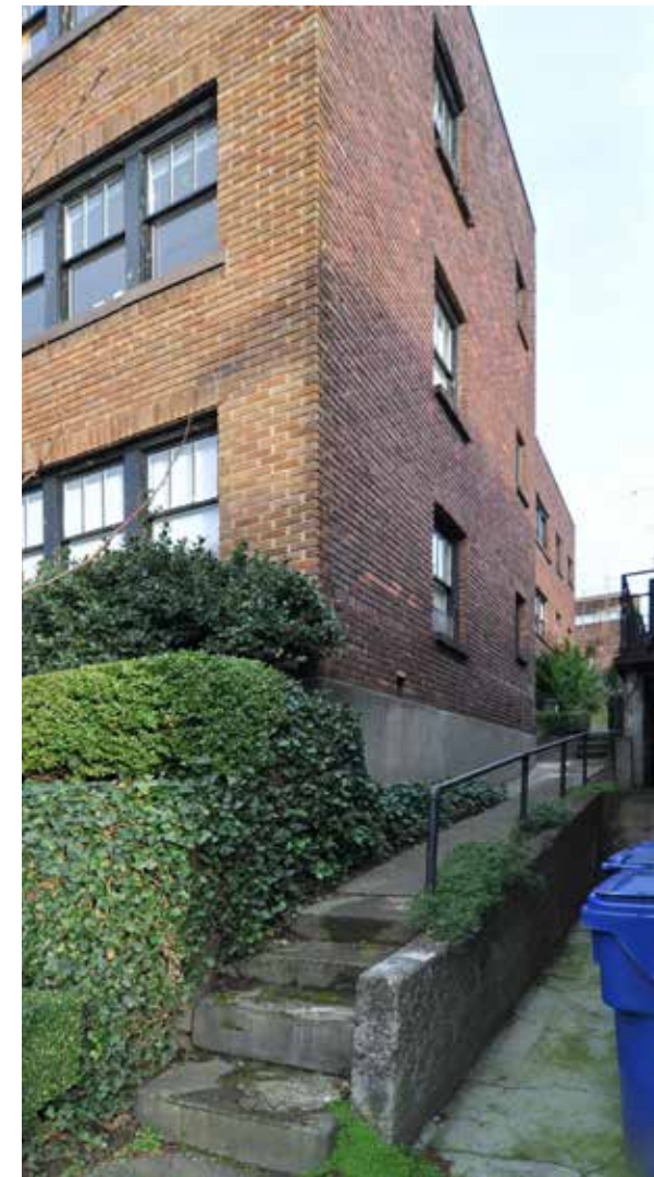
4 View to West of South property line condition
