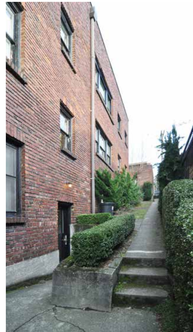
5 View of path through site along south side
