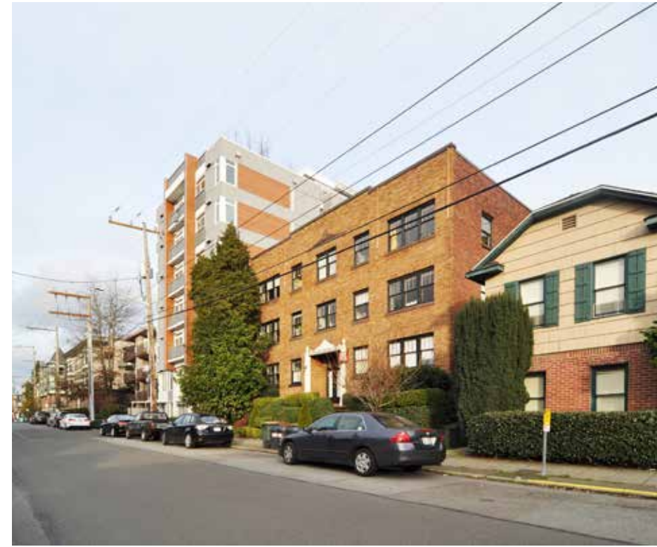
1 View of site looking Northeast on Summit Ave E
