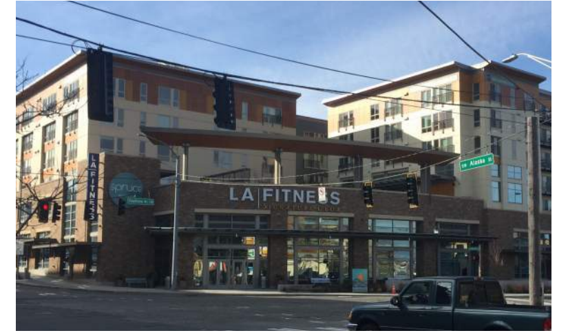
D. ADDRESS: 3900 SW Alaska Street BUILDING/USE: LA Fitness / Multi-Family Housing
