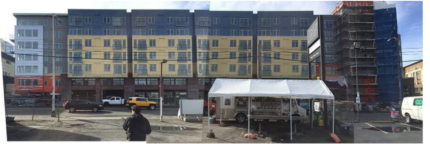
E. ADDRESS: BUILDING/USE: Multi-family Housing (Under Construction)
