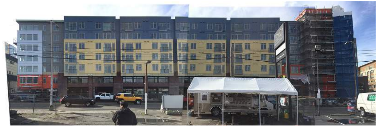
F. ADDRESS: 4755 Fautleroy Way SW BUILDING/USE: Multi-family Housing (Under Construction)
