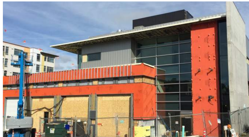
H. ADDRESS: BUILDING/USE: Fire Station (Under Construction)
