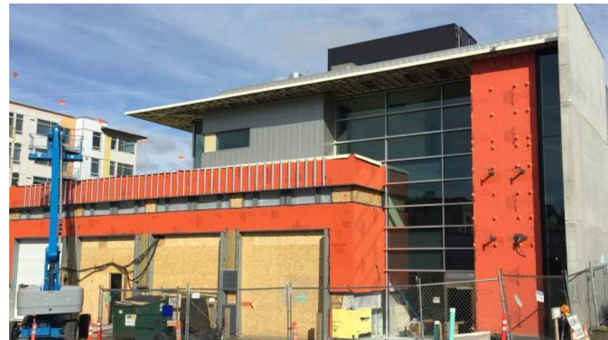
H. ADDRESS: 3715 SW Alaska Street BUILDING/USE: Fire Station (Under Construction)
