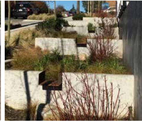
Bioretention Planter Wall
