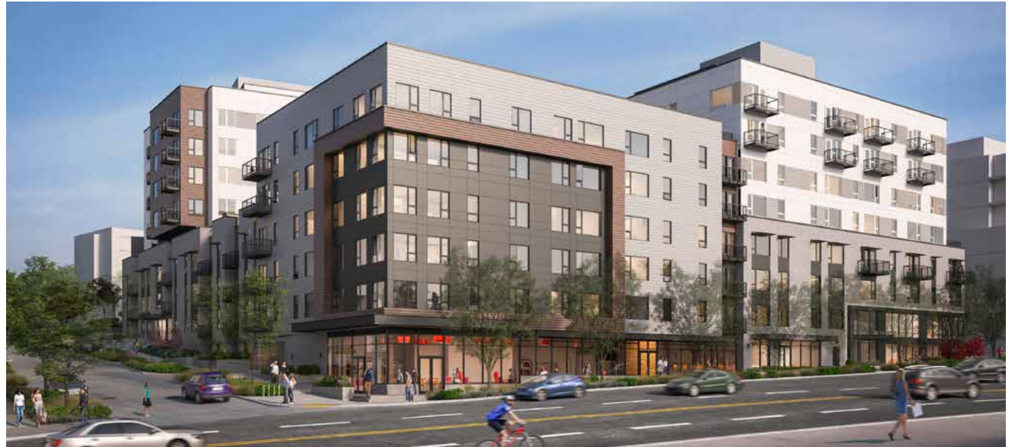
VIEW FROM SE CORNER
