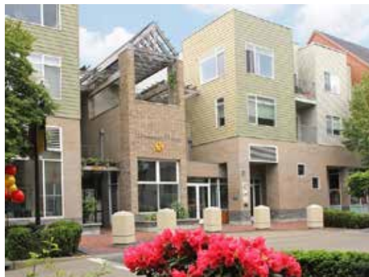
CMU + aluminum storefront base, fiber cement above
