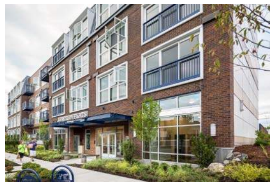
④ JUNCTION FLATS APARTMENTS
