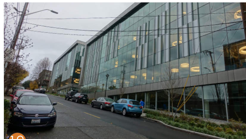
12 looking NE at 3rd Ave. W
