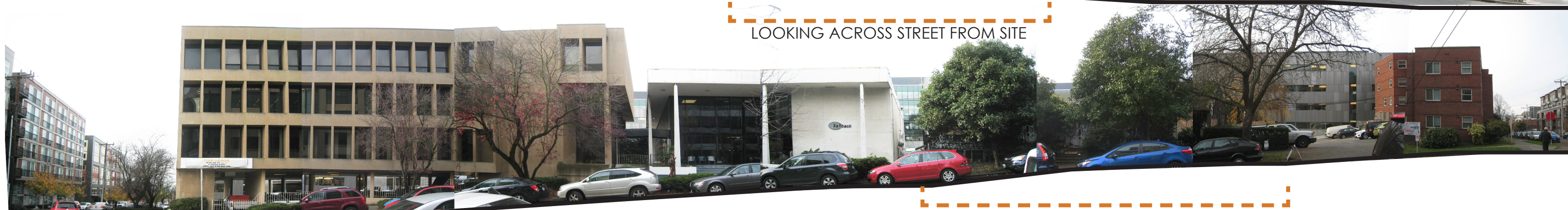
4 Looking West across 2nd Ave. W
