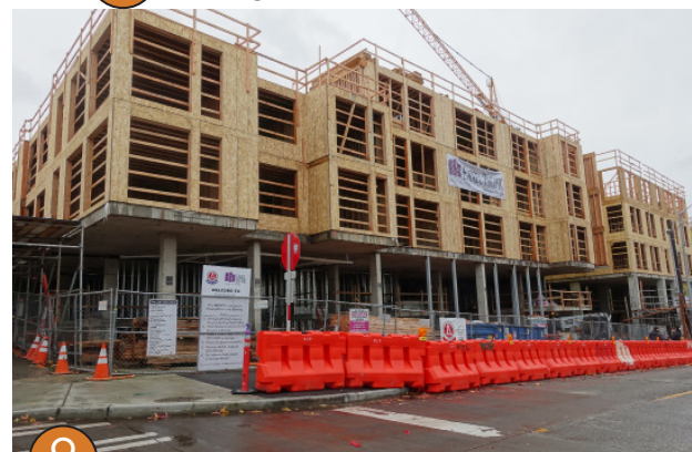
9 looking SE at Harrison St.
