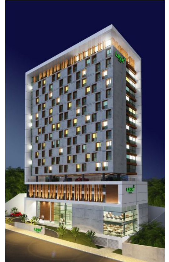
Frame around building edge
