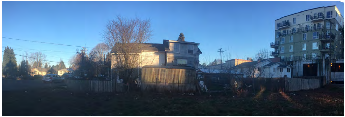
3 NORTH PROPERTY LINE LOOKING NORTH
