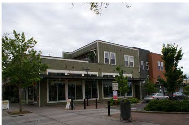
9 Morrow Lane Looking Southwest - Phase II 1-Way Private Through-Block Connection 2-Story Commercial Building
