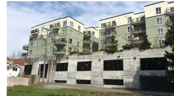
8 TOWERS ON GREENWOOD FROM ALLEY
