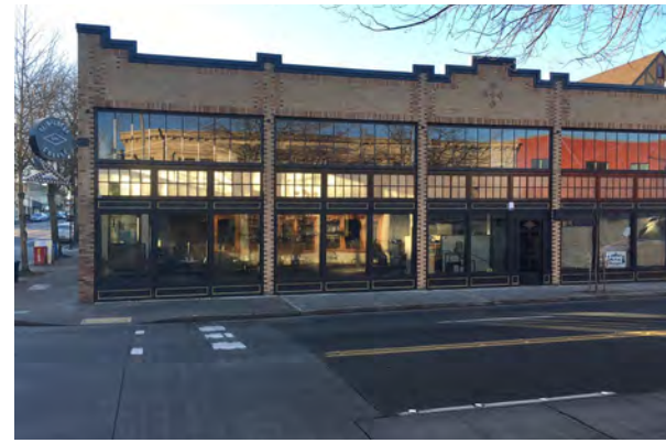
7 Flintcreek Cattle - Greenwood Storefront
