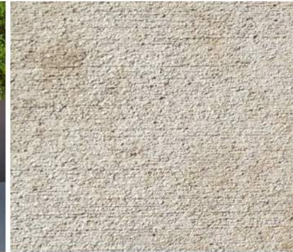
CONCRETE TOPPING SLAB AT PET AREA
