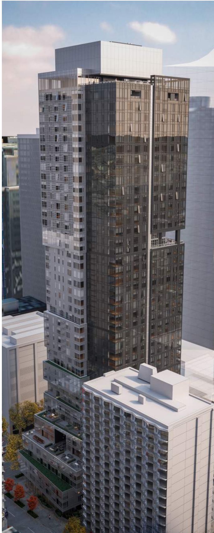
VIEW FROM NW CORNER
