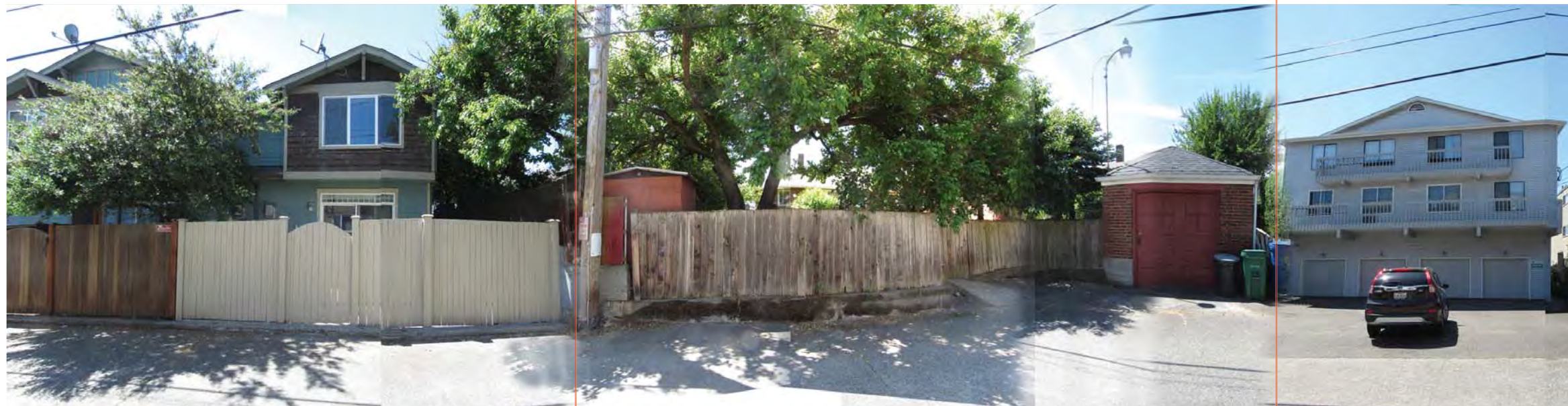
PROJECT SITE EXISTING STRUCTURES TO BE DEMOLISHED
