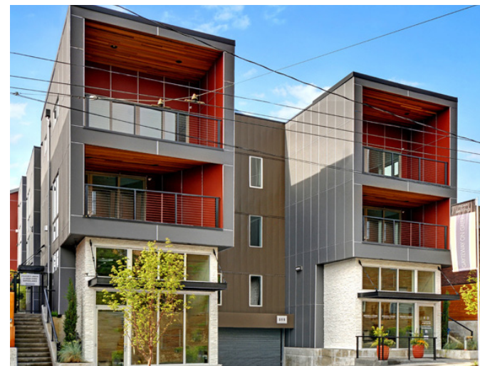
Galer 8 by NK Architects
